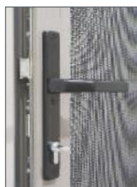
Center Latch, Lock and Handle of the Multi-Point Security Latching System
