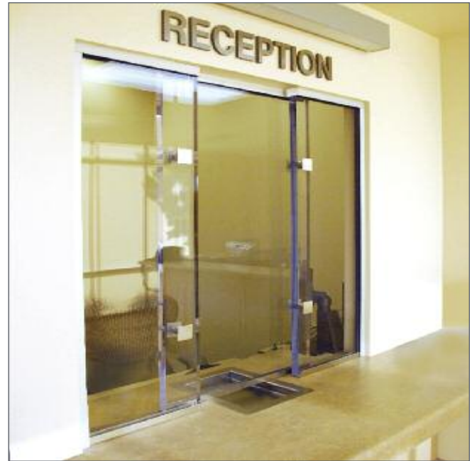
Typical Bullet Resistant Barrier with Snap Together Sash on Top and 1-1/4" (32 mm) Aluminum U-Channel on Bottom
