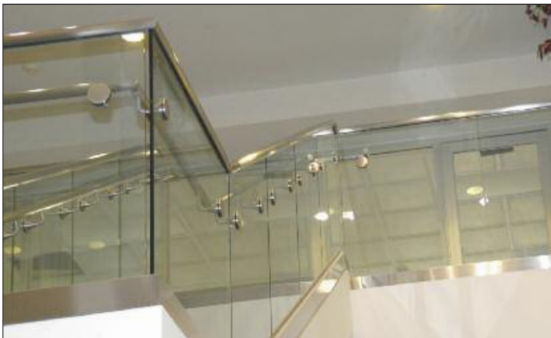
System: TAPER-LOC® Glass Railing With 2" (51 mm) Top Cap and 1-1/2" (38 mm) Hand Rail
