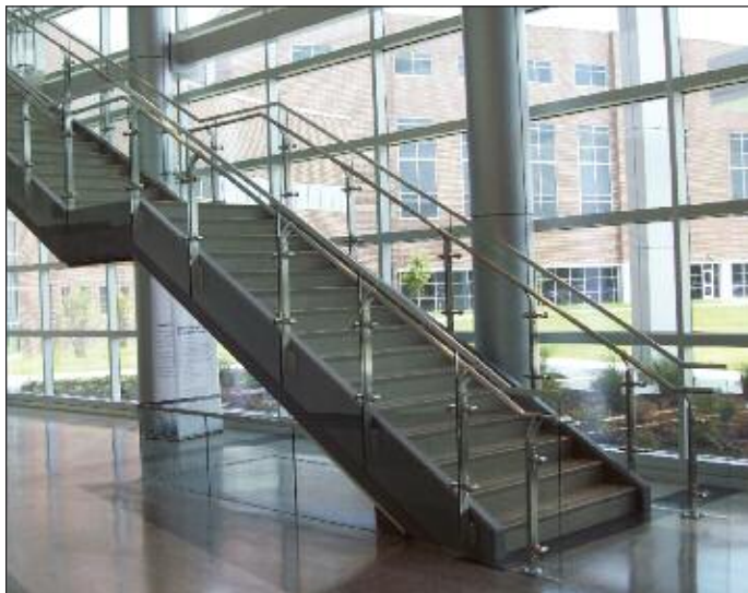
System: P2 Series Fascia Mount Post Railing With Glass Infill
