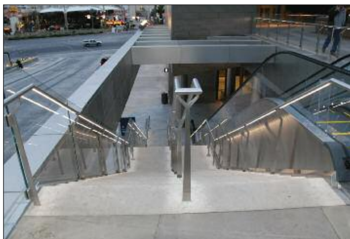
LED Light Strips in CRL Hand Railing installed at CityCenter, Las Vegas
