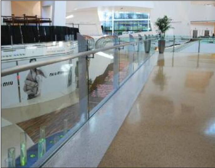
System: TAPER-LOC® Glass Railing With 2" (51 mm) Hand Rail
