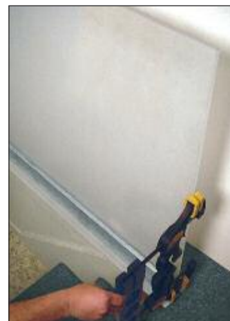
STEP 4: Turn adjustment knob on the Clamp and Alignment Fixture until the glass is plumb.
