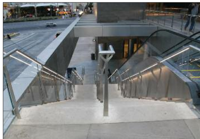
LED Light Strips in CRL Hand Railing Installed at Stair Locations (See pages 373B-377B for Hand Rail LED Information)
