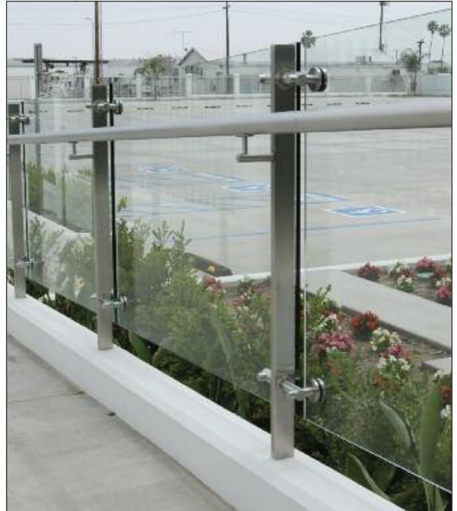
System: P3 Series Stainless Steel Railing With 1-1/2" (38 mm) Hand Rail
