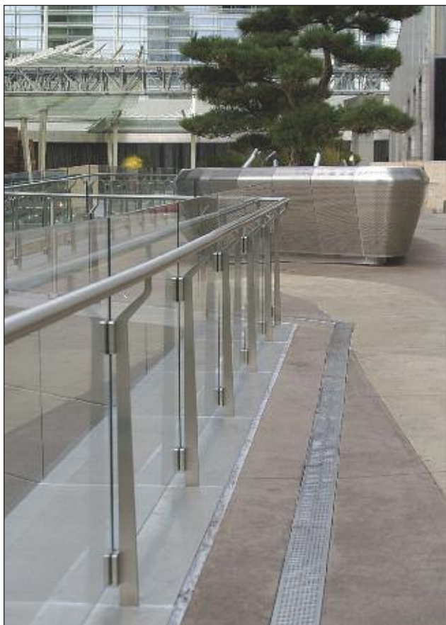
System: Custom P5 Series Post Railing With Glass Infill
