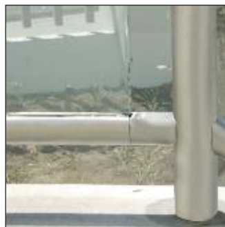
Field measure to next Rail Adapter for accurate cut length on Bottom Rail
