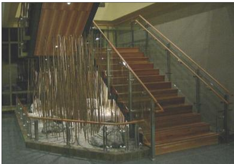
System: P8 Series Post Railing With Glass Infill
