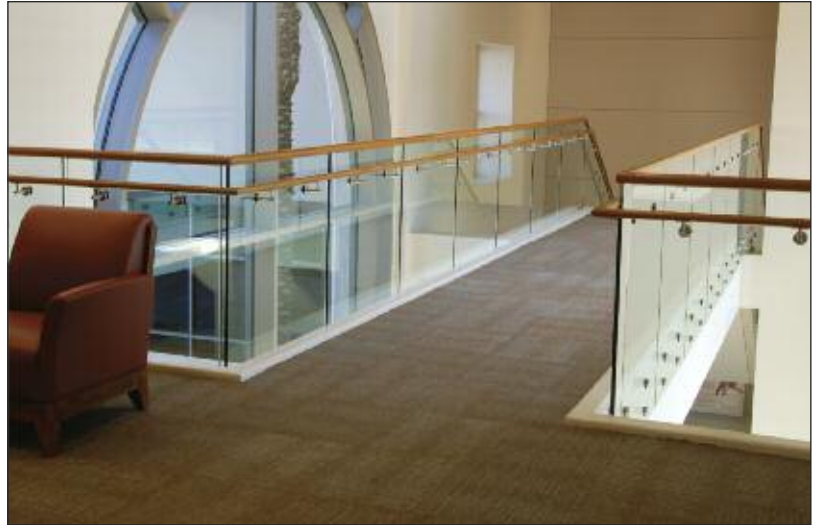
System: SRS Standoff Glass Railing With 2" (51 mm) Wood Top Cap and 1-1/2" (38 mm) Hand Rail.
