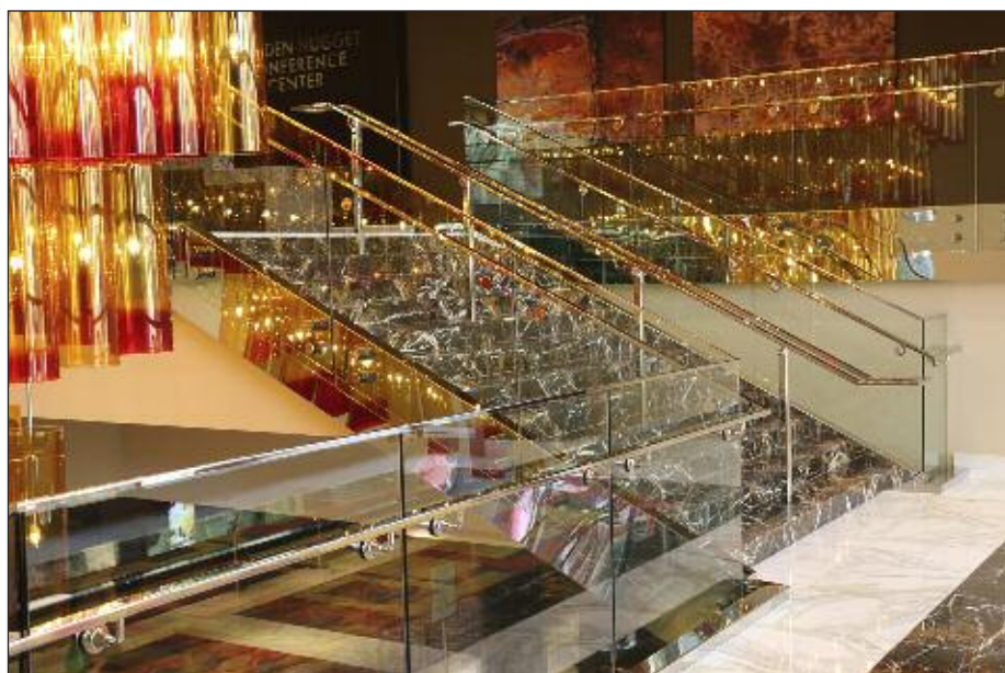
1.9" (48 mm) Hand Rail With Newport Series Glass Mounted Brackets
