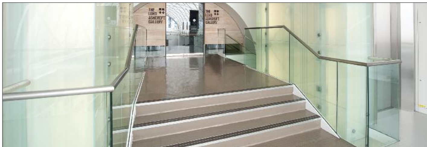
System: TAPER-LOC® GRS Glass Rail With 2-1/2" (63 mm) Top Cap
