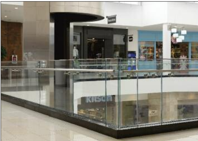
System: TAPER-LOC® Glass Railing With U-Channel Top Cap and 2" (51 mm) Hand Rail
