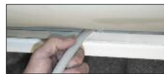
STEP 5: Pour in Expanding Cement to 3/8" (10 mm) below the top. Allow adequate time for it to set.
