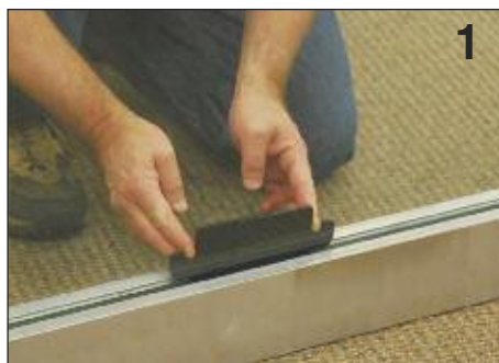
Place the TAPER-LOC® Tapers into Base Shoe finger tight at designated spacing.
