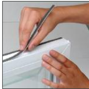
Remove old Pile from frame
