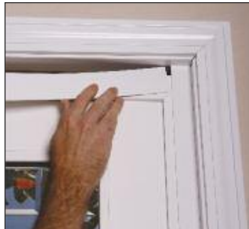
3. Add Flat Trim to Fill Gap Between Jamb and Frame
