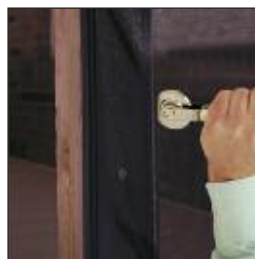
3. Roll in screen wire and retainer spline
