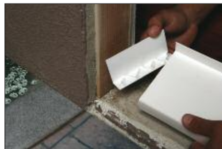
Apply VL21 "L" Shape with M64 Polyurethane Sealant
