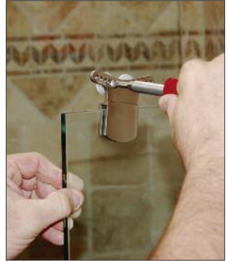
Adjusting a Sagging Door
