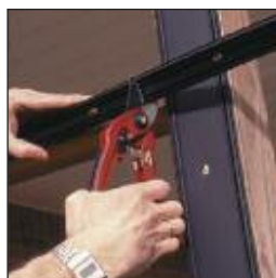
1. Measure and cut Screen Tight Base
