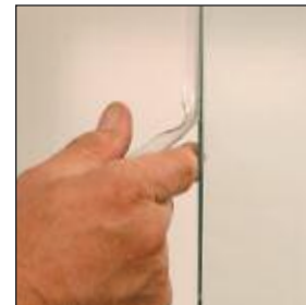
Remove the damaged or brittle water seals.
