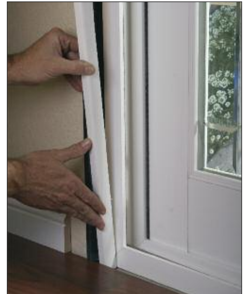
Vinyl Stop Used as a Jamb Extender
