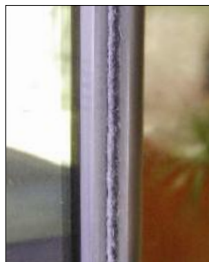
Press new pile into groove with screwdriver
