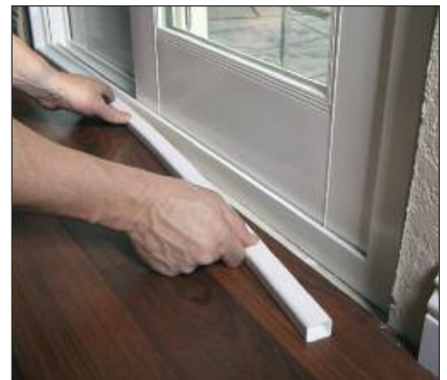
Vinyl Stop Used as a Base Shoe to Cover Gap
