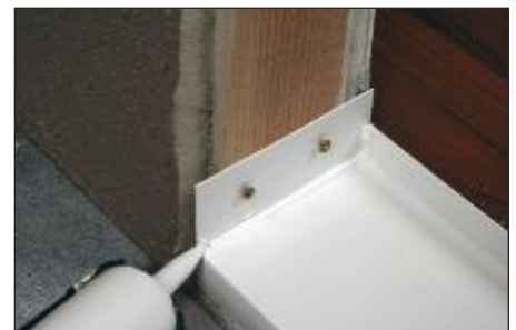
Fasten Sill Pan to Wall and Seal Seam
