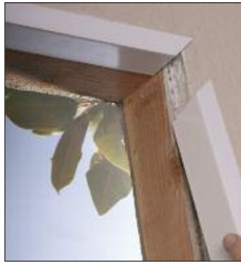
1. Add L-Shape to Cover Jamb and Drywall
