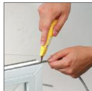
Cut to length with knife or scissors
