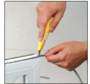
Cut to length with knife or scissors
