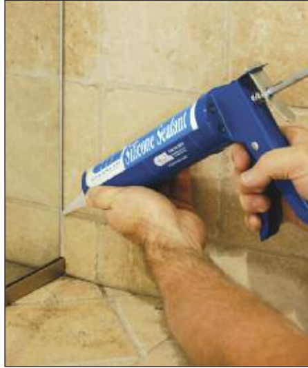
Resealing a Leaking Unit
