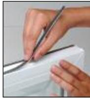
Remove old pile from frame
