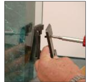
Replace with new gasket, interior cover plate, and screws, then secure in place.
