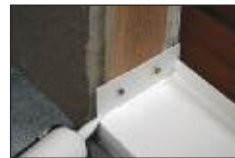
Fasten Sill Pan to Wall and Seal Seam
