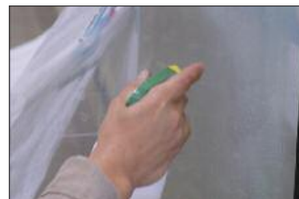
Spray Solution on Adhesive
