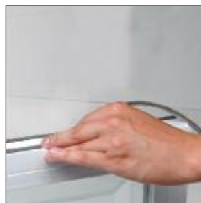
Press new Zipper Pile into groove with finger
