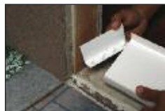
Apply VL21 "L" Shape with M66 Polyurethane Sealant
