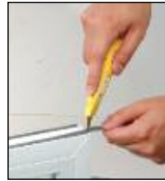
Cut to length with knife or scissors
