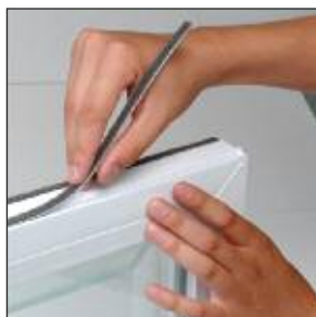
Remove old Pile from frame
