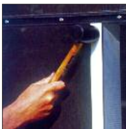
4. Snap on Screen Tight Cap
