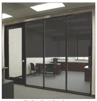
Offset Glazing Allows for Window Coverings
