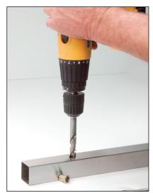
First, drill the appropriate size hole for the Rivet-Nut into your round post or square tube
