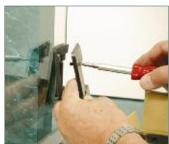
Install a new gasket and interior cover plate, replace screws, then secure in place.
