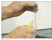
Cut the new and matching water seals to the same length as the originals and install.
