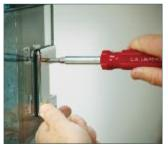
After alignment, tighten the cover plate screws by hand. Do not use a power tool, or you risk damaging the screw heads
