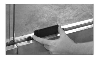
Step 2 Use the TLK12 Installation/Removal Tool to push the Tapers down into position for the next step, locking the Tapers together.
