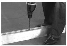
Step 2 Clean out the holes with CRL's Blow Out Pump Cat. No. EBADP1.
