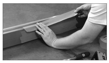
Step 4 Complete the process by removing the Tapers from the Base Shoe, then adjust or replace the panel.
