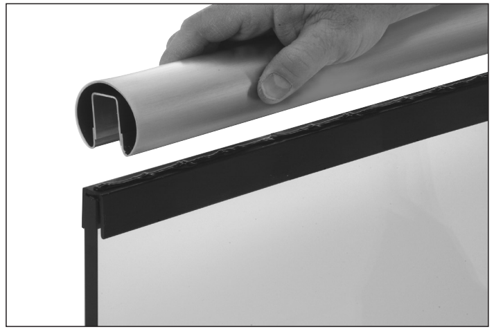
Install the Cap Rail over the Silicone and Protective Vinyl Insert.
