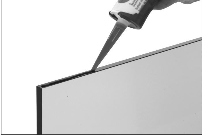
Apply Structural Silicone to the top edge of the glass.
