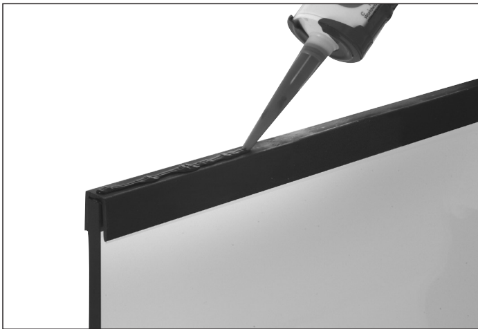
Apply Silicone to the top edge of the Protective Vinyl Insert.
